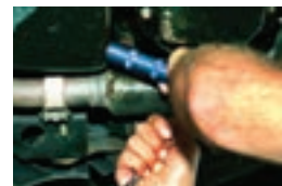
TAPPING DRAIN HOLE
