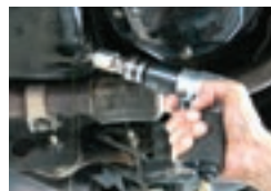
DRILLING DRAIN HOLE
